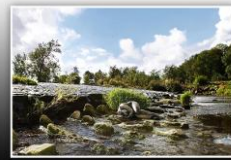
WEIR Ort: Gronau Location: Leine-Wehr Model: Alexandra
